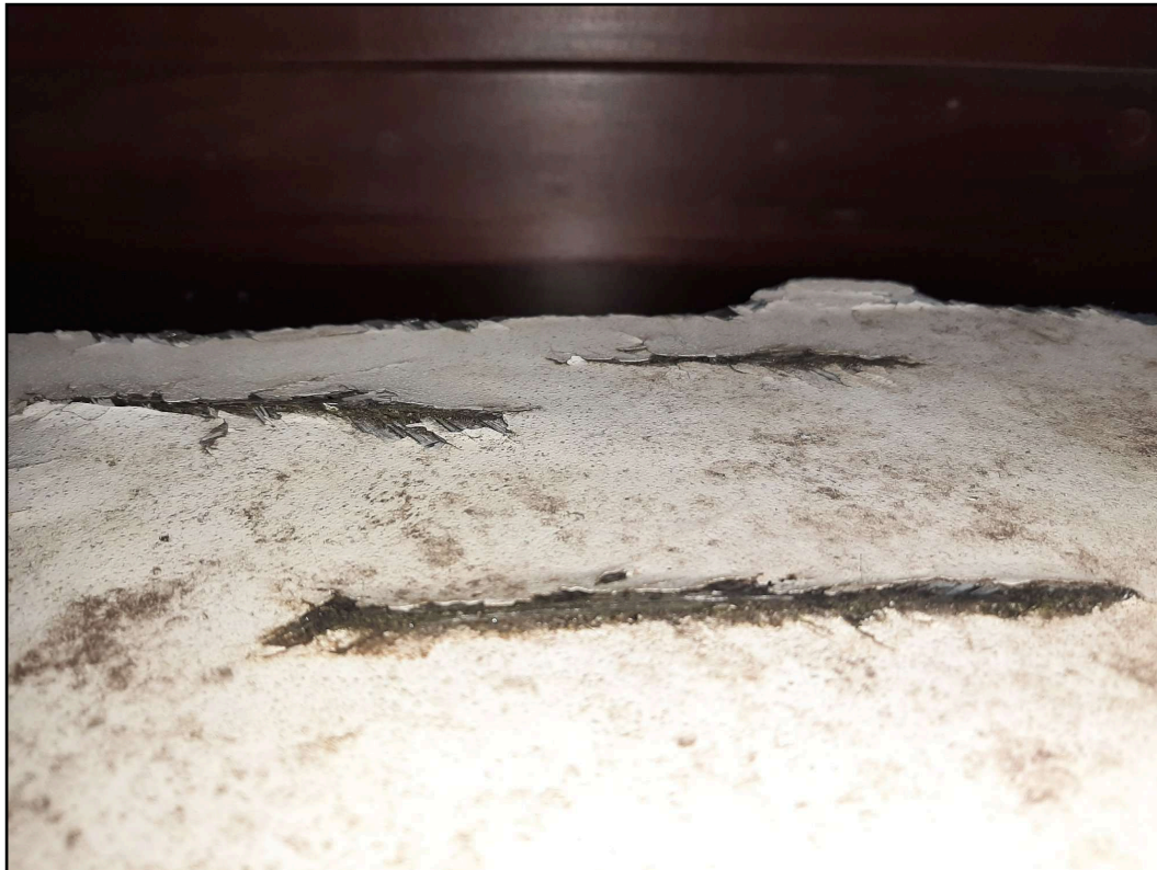
Figure 29: Close up of the lifting of the surface of the white side.
