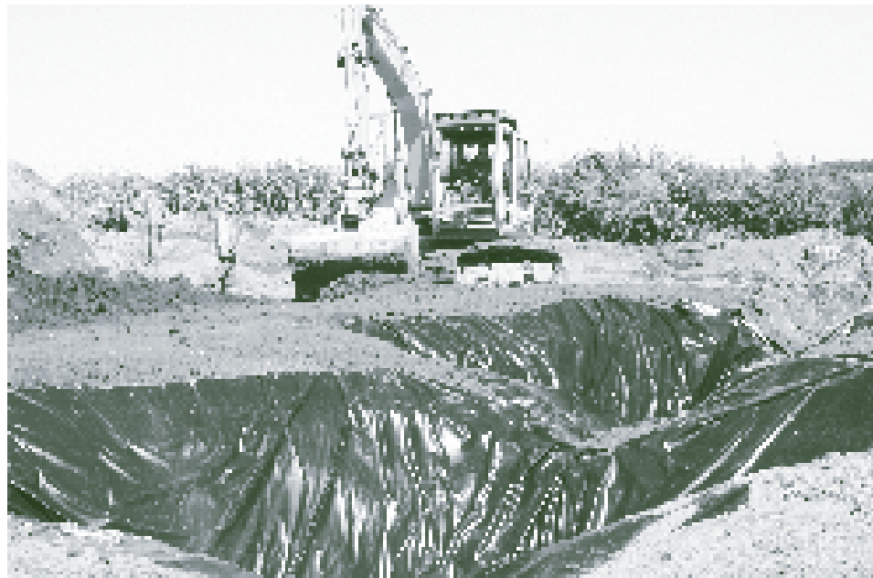
Figure 5.2 Construction of a flare pit at TAG Oil's Cheal-C well site in Taranaki. The clearly visible plastic lining is designed to prevent contaminants from leaking into soil and groundwater.
