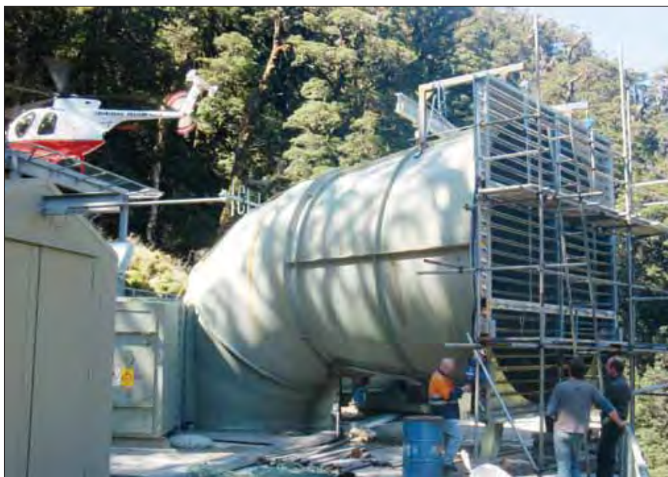
Figure 8.7: Easé showing louvres being installed
