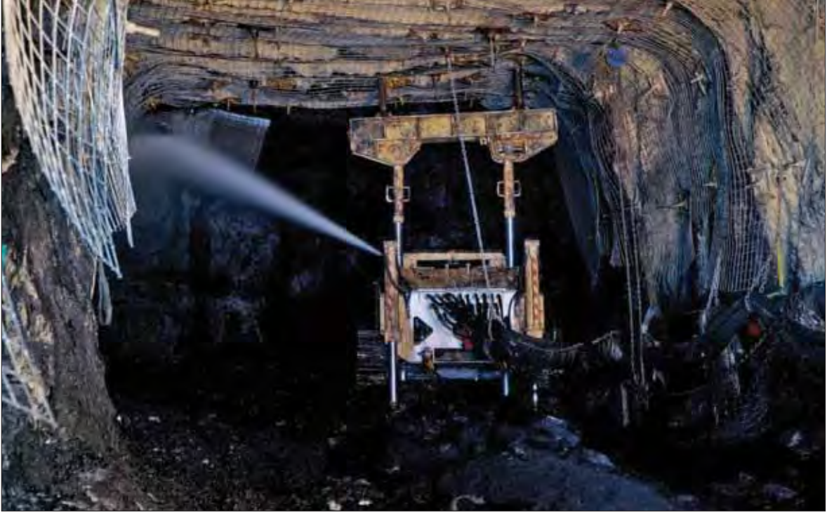
Figure 12.2: Hydro monitor at work 3
