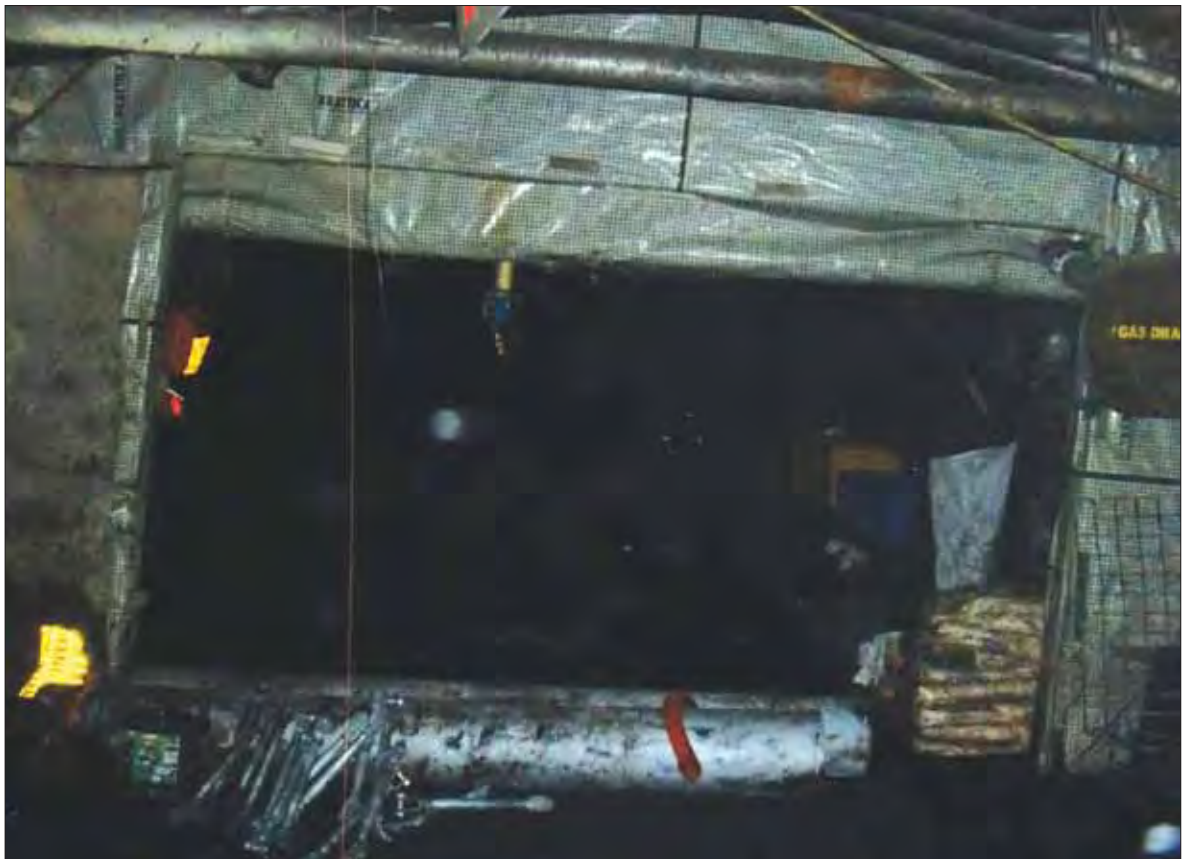
Figure 16.3: View of the upper FAB looking inside 79
