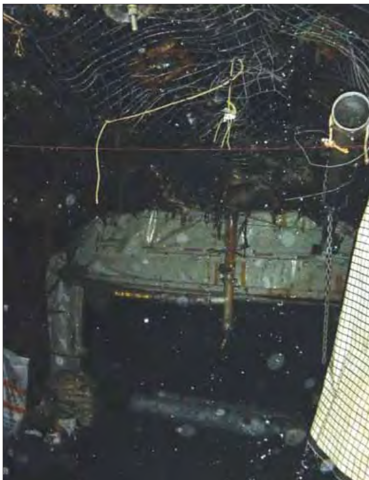
Figure 16.4: Inside the upper FAB looking towards the entrance 80
